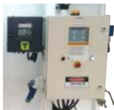
Portable Fuel Station fuel management system and electrical control box with emergency stop
