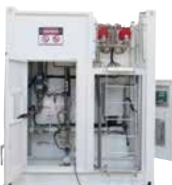
Bulk Storage Easy access to pump bay, man-way and dipping points
